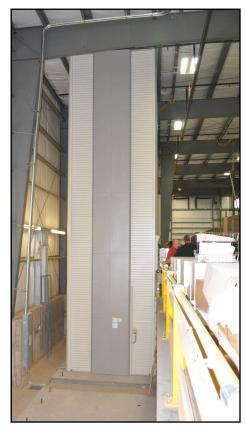
By placing the Lean-Lift into a speciallyconstructed below-grade pit, a taller unit with more storage could be used.
